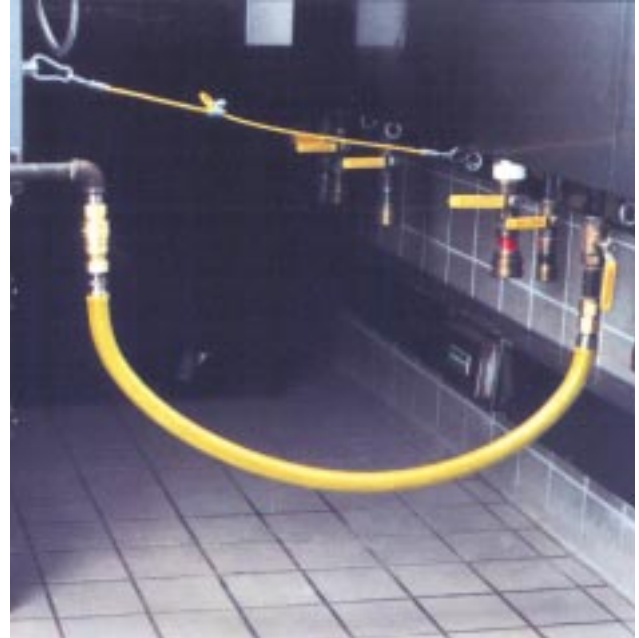
Flexible gas quick connectors enable the operator to move appliances more easily for cleaning behind the cooking line.
